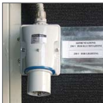
▲ Auxiliary supply connection, 220-240VAC Raccordement auxiliaire d'alimentation, 220-240VAC
