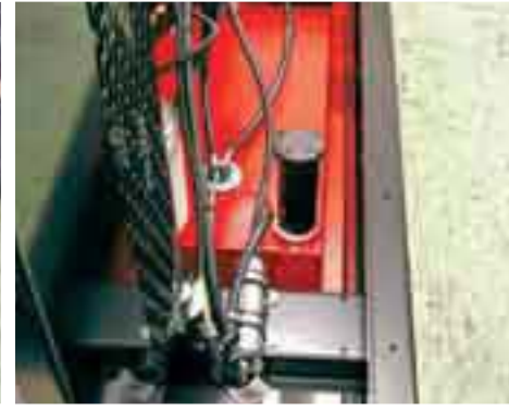
🔍 Bunded base system for engine liquids, fuel leaks and acids Bac de rétention liquides moteur, carburant, acide batterie
